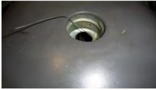
**4.** Use a small piece of electrical tape to securely attach the ends of the sensor wires to the Mechanic's Wire.
