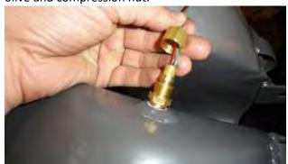
10. Ensure that the sensor is in the correct position with the circlip lightly resting on the inside of the tank before tightening the compression nut, as the olive is one-time-use and cannot be removed and installed again. Use a 9/16-inch wrench to tighten the compression nut until it starts to crush the olive, then tighten an additional 1/3 turn to create the seal.
